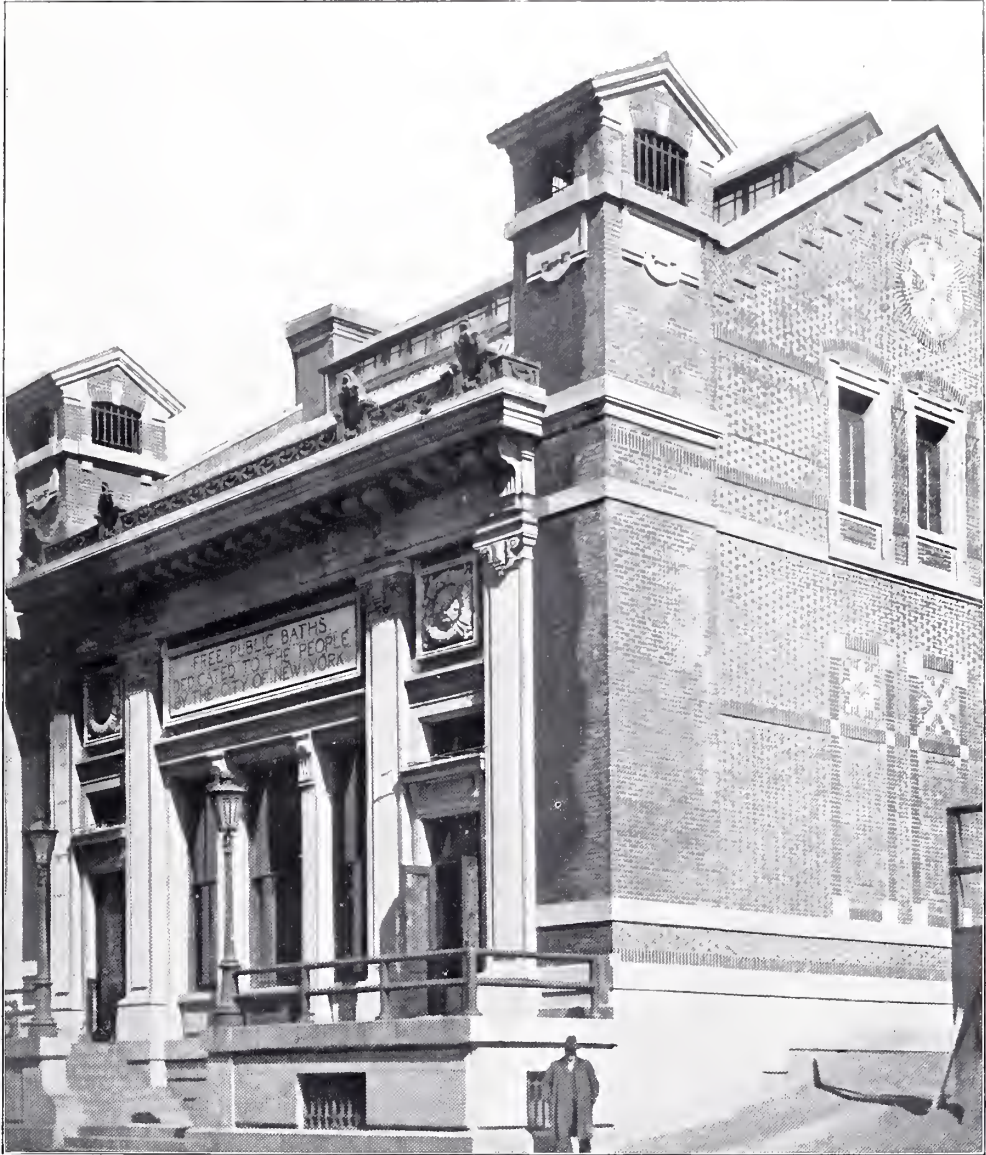
Free Public Baths, John Jay Park, East 76th Street, New York City, STOUGHTON AND STOUGHTON, Architects.
